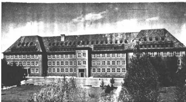
GOSSEN MAIN FACTORY
